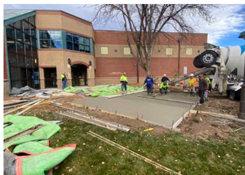
Chilson Recreation Center entryway improvements under construction
