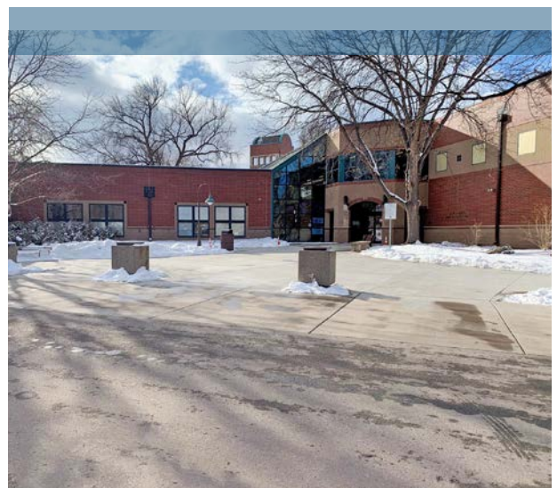
The completed Chilson main entrance ADA compliance project
