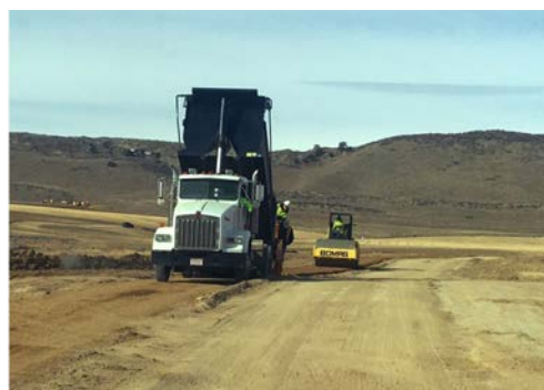
Construction at Prairie Ridge Natural Area
